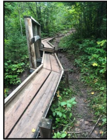
Examples of worn-out trail and failed built structures that must be replaced for user safety and erosion concerns.
