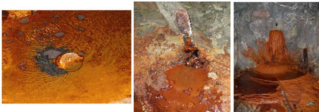
**Fig. 1.** Representative boreholes on level 27 of the Soudan Iron Mine. Left and middle images are vertical boreholes found in the west tunnel while the right image is of a horizontal borehole drilled in the east tunnel.
