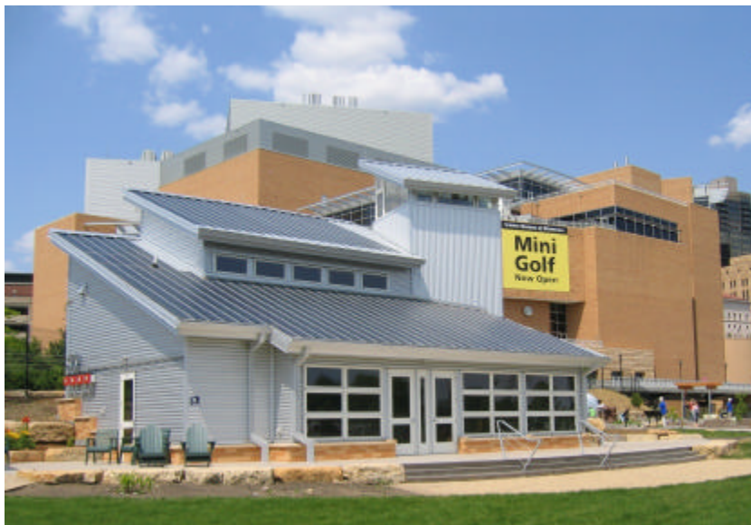
This 1,200 sq. ft. Science House uses a photovoltaic (solar) roof and ground-source heating and cooling systems to provide all the energy it needs to heat, cool, and power itself on an annual basis.
